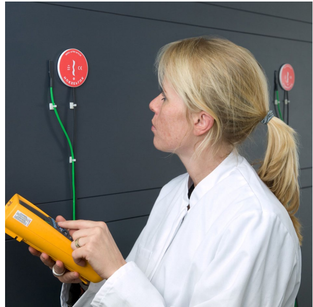
Figure 1 On-site measurement of building envelope thermal resistance
