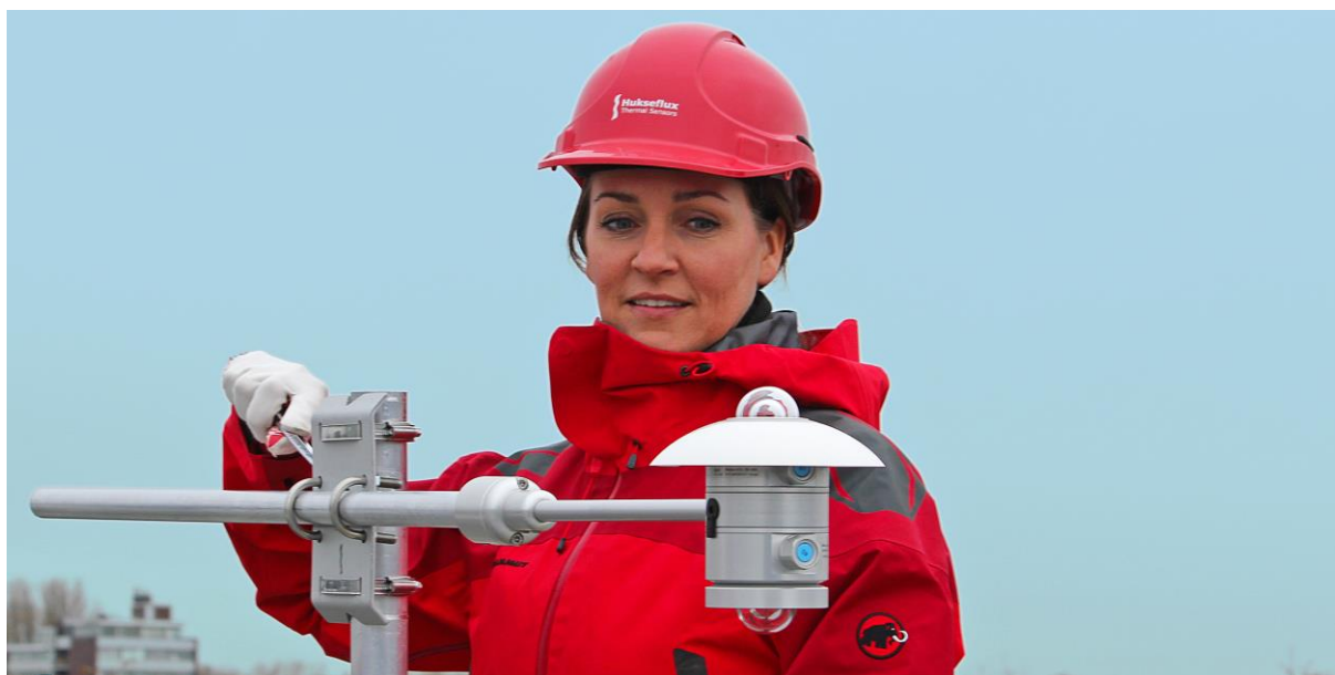
Figure 0.1 An albedometer being installed with its rod mounted securely to a mast thanks to ALF01 levelling fixture and CMF01 crossarm mounting fixture
