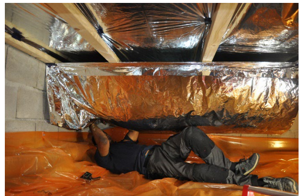
Figure 2 TONZON's thermal cushions significantly reduce heat loss and ensure thermal comfort through warmer floors and heat retention.
