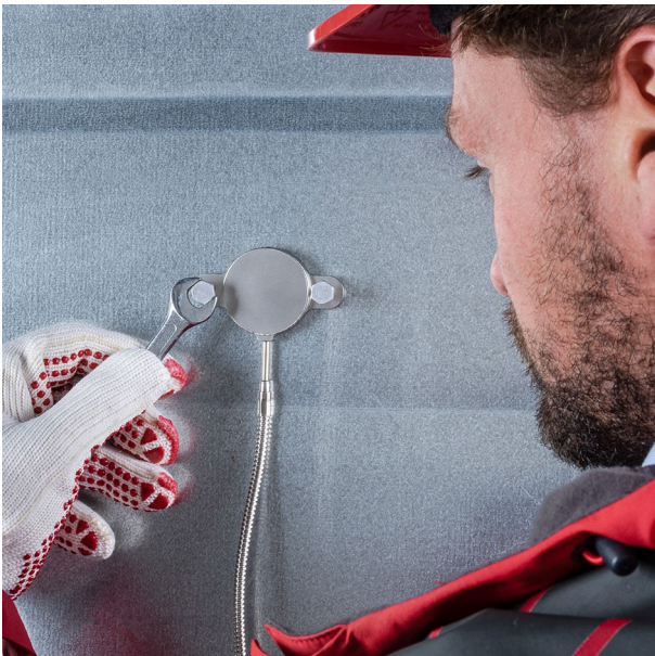
Figure 4 IHF02 industrial heat flux sensor bolted to the surface. Note that the optical properties of sensor and surrounding metal are matching (both blank metal). Springs are not visible.
