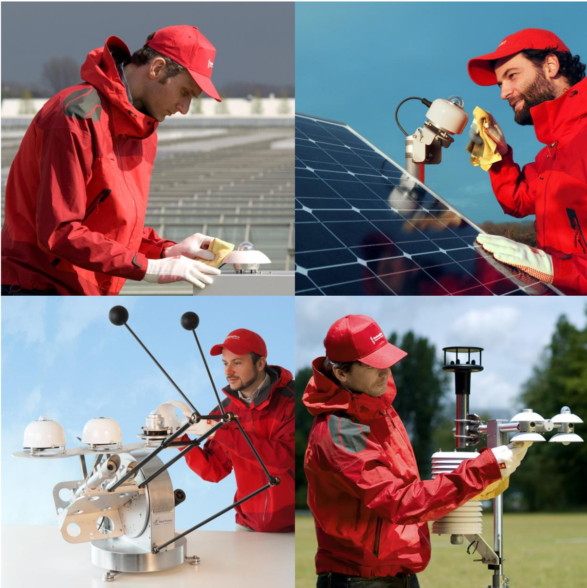
Figure 2 Examples of solar radiation measurement installations, a) Global Horizontal Irradiance b) Plane Of Array irradiance c) complete solar measurement system with separate measurements of Direct Normal Irradiance, Global Horizontal Irradiance, Diffuse Horizontal Irradiance and longwave radiation d) A meteorological station with a measurement of net radiation using a 4-component net radiometer.
