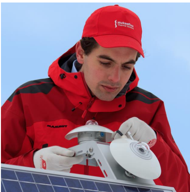
Figure 2 dual setup in PV system performance monitoring
